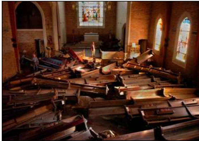
St. Paul's Church after the destruction from Hurricane Katrina.
